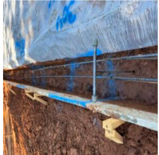
Left half of rear footing probed soft
