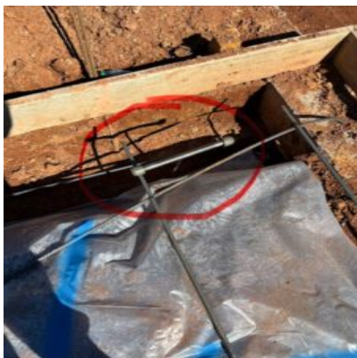
Red line indicates loose fill along sub wall left side
