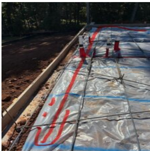
Red line indicates loose fill along sub wall left side
