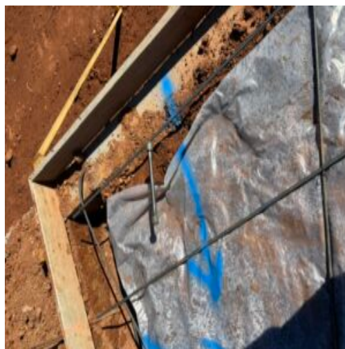
Probing loose backfill along sub wall
