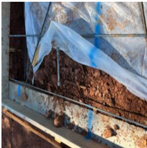
Probing loose backfill at sub wall
