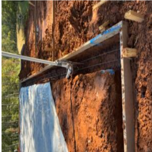
Right side exterior footing and slab
