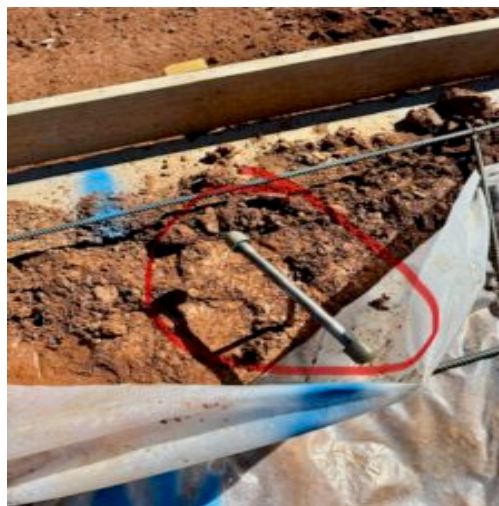
Probing loose backfill along sub wall
