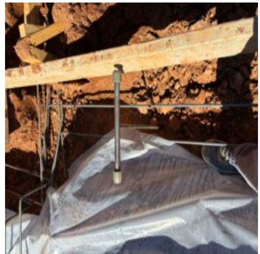
Left half of rear footing probed soft
