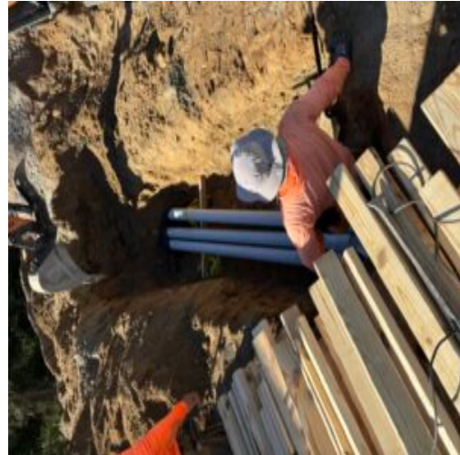
Moving electrical conduits outside curb west side of bridge abutment
