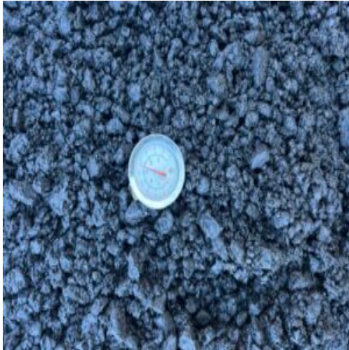
Temperature checks on hot mix
