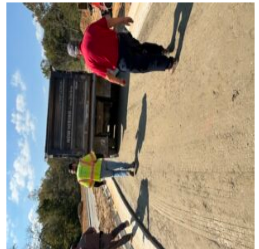
Proof rolling of subbase using a loaded tandem dump truck having 17.95 tons at both sides of bridge.
