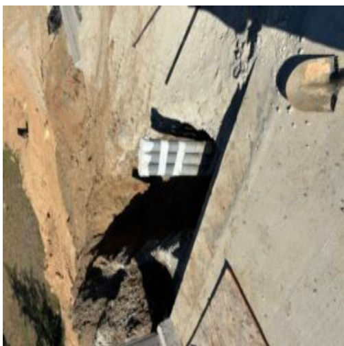
Moving electrical conduits out side of curb area at bridge abutment
