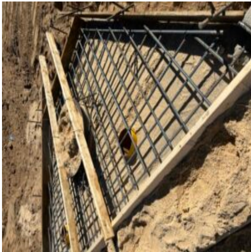
Reinforcing observed at Unit 4 phase 2 throats
