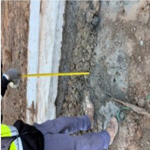
Observing subgrade depth at roundabout
