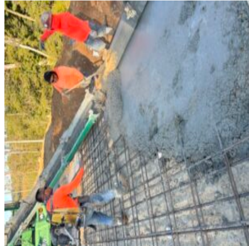
Concrete placement at west side bridge approach slab.
