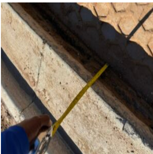
Observation of subgrade prep. at Unit 4 phase 2
