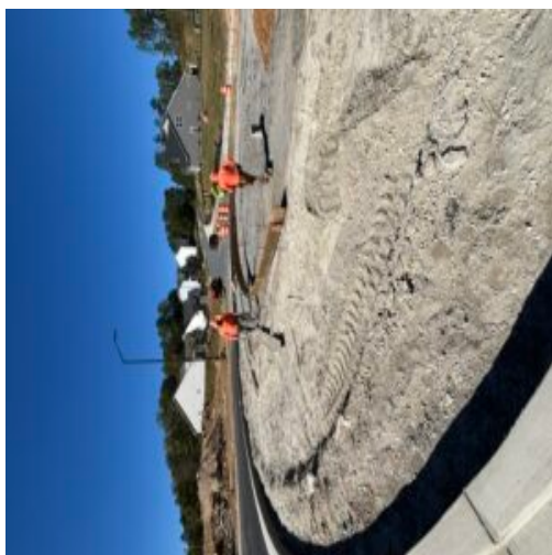
Subbase prep.and forming for outer and inner curb pours.
