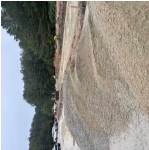
Subbase prep.for curbing pour at exit drive east side of bridge abutment
