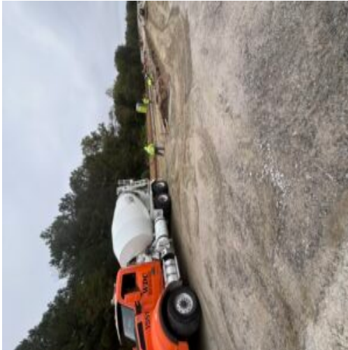
Pouring curbing at exit drive from east side bridge abutment
