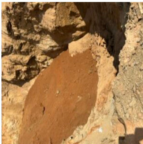
Fill soils being placed back into excavated borrow pit #2 south of building lot # 24
