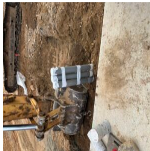
Backfilling at electrical conduits holes at bridge abutments.
