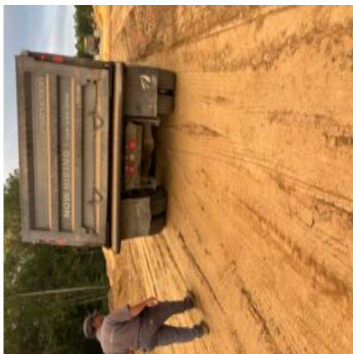
Observing proof rolling of subgrade at Nature Walk Pkwy. between sanitary sewer manhole #3 and #2
