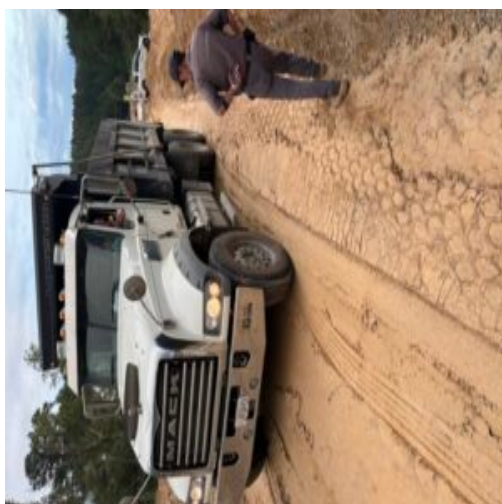
Observing proof rolling of subgrade at Nature Walk Pkwy. between sanitary sewer manhole #3 and #2
