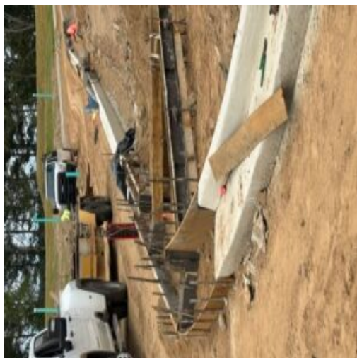
Curbing poured at Unit 4 phase 2
