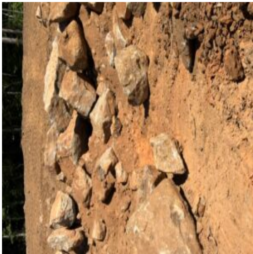
Rockfill was stopped to correct placement procedures lot #25
