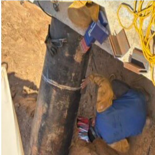
Pushing 24" casing welding sections
