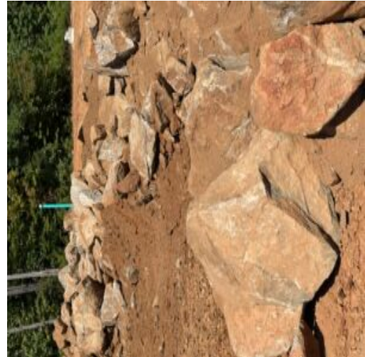
Rockfill placement is not in compliance
