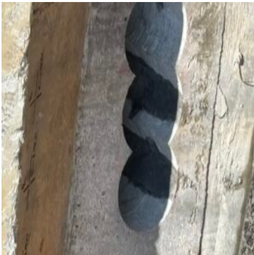
6" core holes cut at bridge for electrical conduits installation
