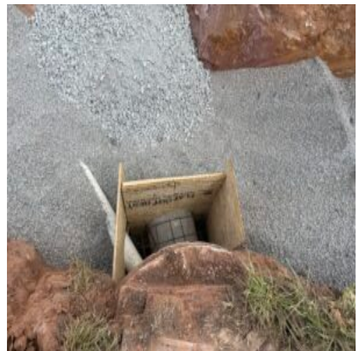
Wire applied around pipe C
