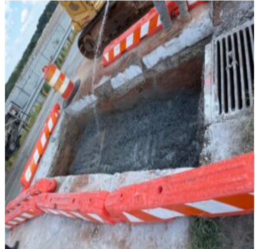
Applying water to GAB
