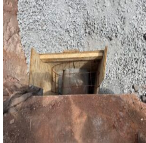
Wire applied around pipe b
