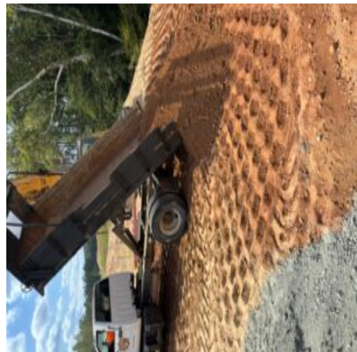
Backfill at west side bridge abutment for sanitary sewer installation to manhole #2
