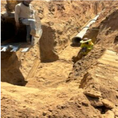
Installation of 18" rcp storm between B6 and B8
