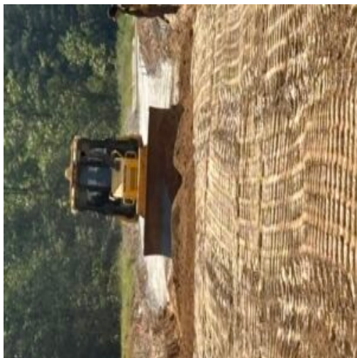
Fill placement and density tests performed at Seven Hills phase 13
