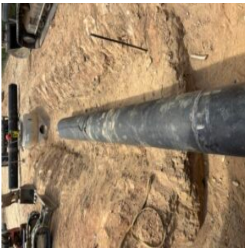
Pushing 24" welded steel casing through opening at bridge for sanitary sewer line.
