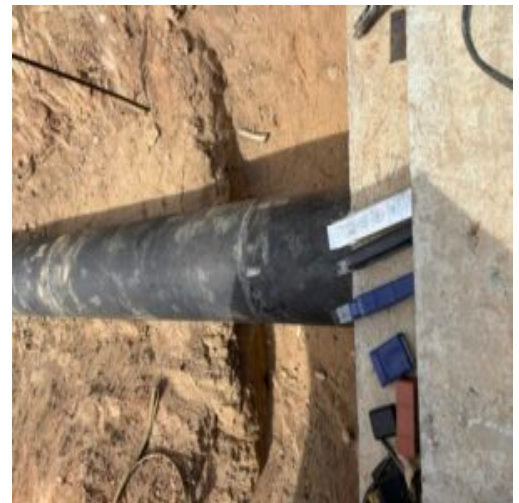
Pushing 24" welded steel casing through opening at bridge for sanitary sewer line.
