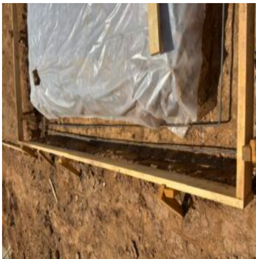
Continuous exterior wall footings
