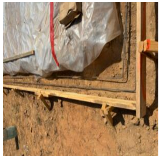
Continuous reinforcing steel in place
