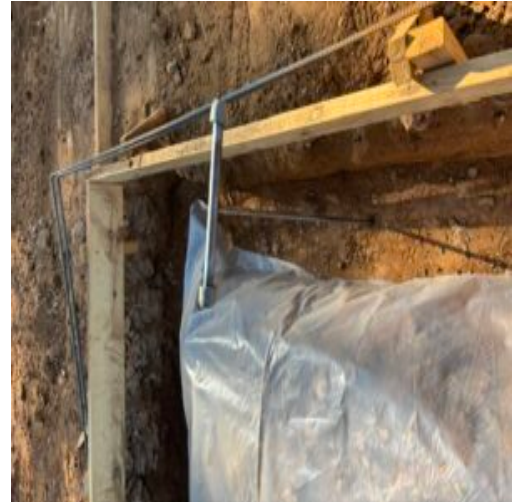
Probing bottom of footings
