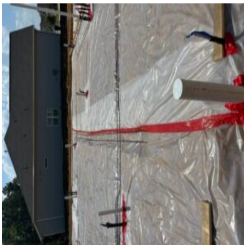
Continuous exterior wall footings
