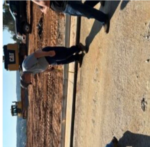
County official checking depth at curb line
