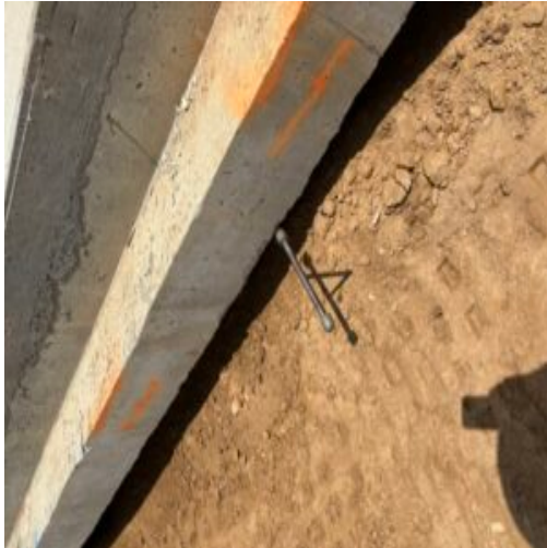
Probing at one foot off wall where it was recommended to use GAB stone
