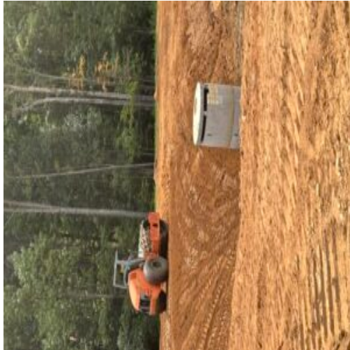
Backfill at Pond A OSC 36" storm pipe
