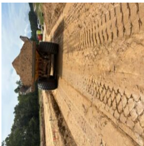
Observing proof rolling of sub grade at Nature walk parkway between sanitary sewer manhole # 3 and 2 using a off road rock truck.
