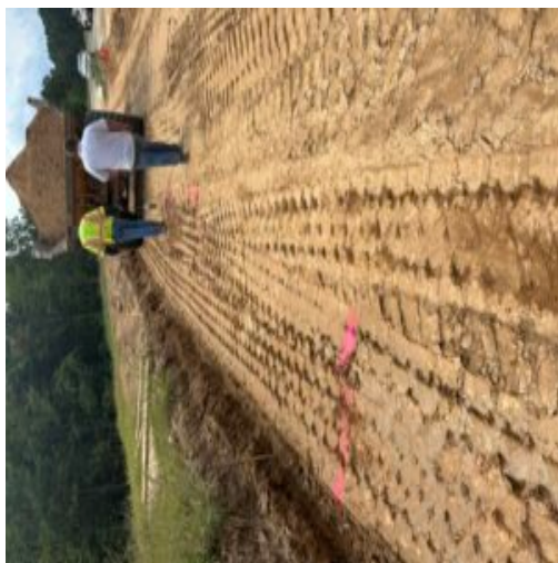
Observing proof rolling of sub grade at Nature walk parkway between sanitary sewer manhole # 3 and 2 using a off road rock truck.
