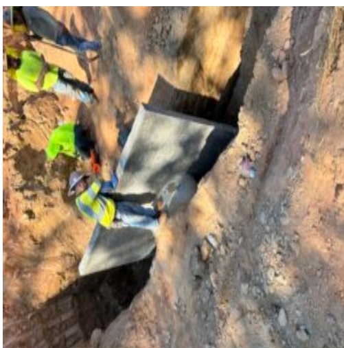
Anti seep collar observed at Pond A
