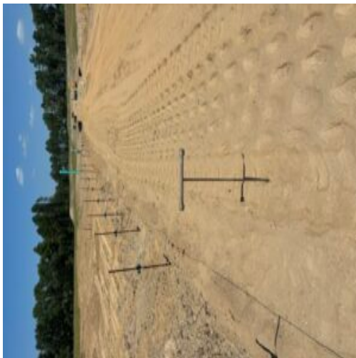
Observation of sub grade for curbing at Unit 4 Phase 2 with recompactng efforts
