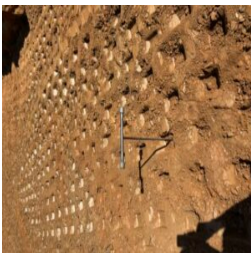
Backfill at Pond A OCS and 36" rcp
