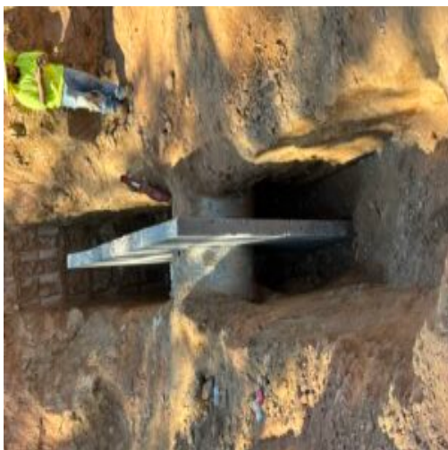
Anti seep collar observed at Pond A
