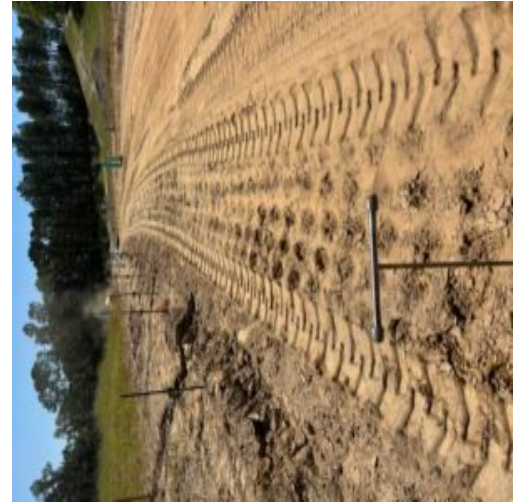
Observation of sub grade for curbing at Unit 4 Phase 2 with recompactng efforts
