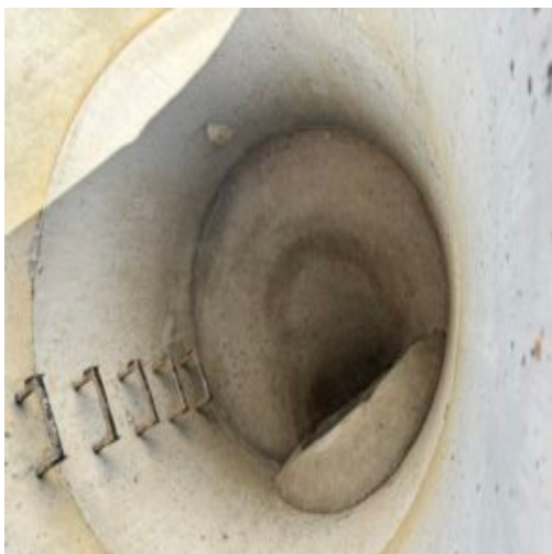
Poured invert at OCS
