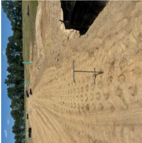
Observation of sub grade for curbing at Unit 4 Phase 2 with recompactng efforts
