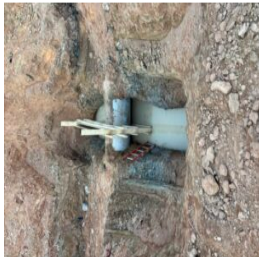
Water at bottom of form work prior to pumping out
