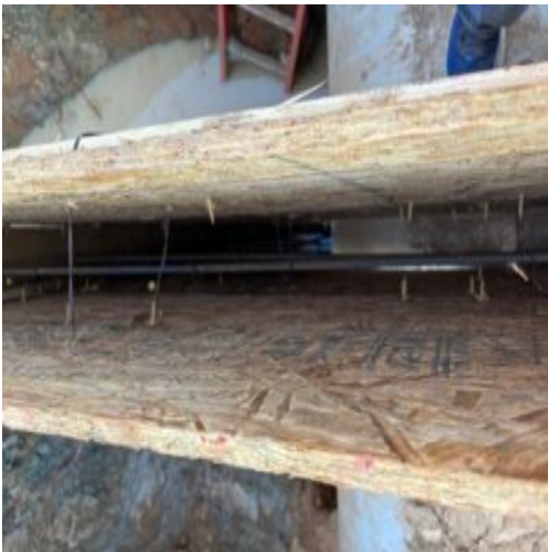
Resteel in form work for anti seep collar
