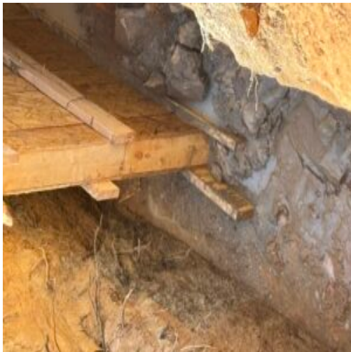
Water pumped out from bottom Of form work
