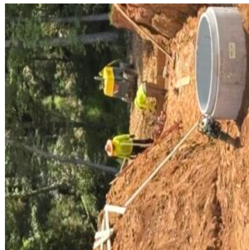
Fill placement and installing anti seep collars
