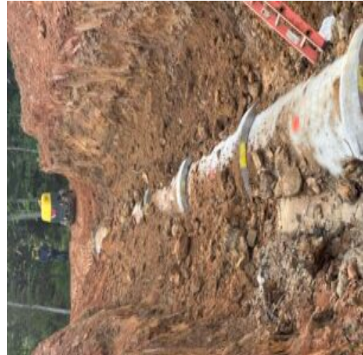
36" rcp installed from headwall to OCS
