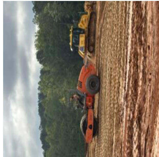
Fill placement at roadway
