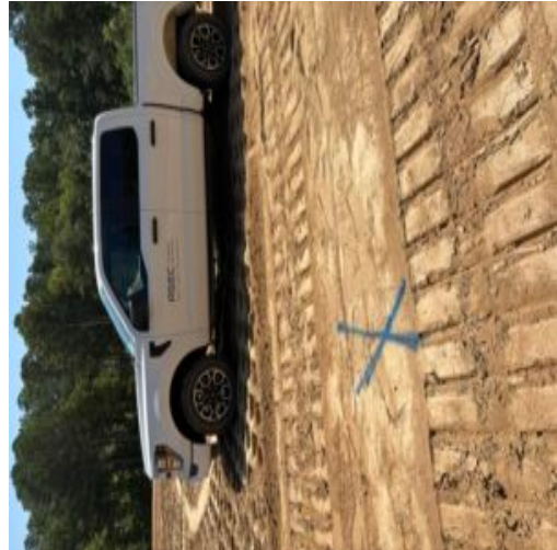
Failed density tests areas with additional compacting efforts recommended
