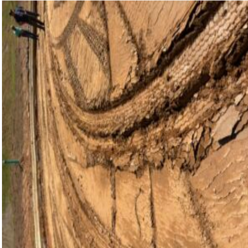
Moderate rutting at cul de sac
