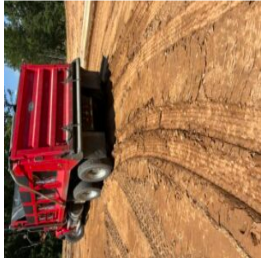
Proof rolling using tandem dump truck with 18.34 tons of base stone
