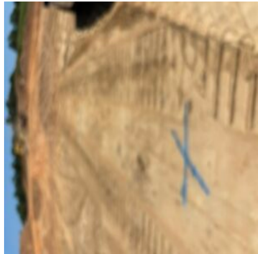
Failed density tests areas with additional compacting efforts recommended
