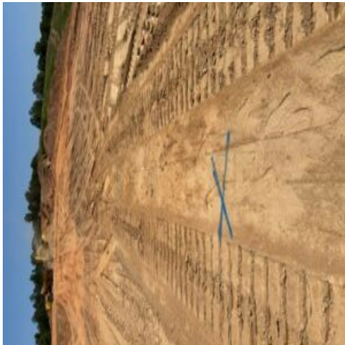
Fill placement at Shelly drive near detention pond
