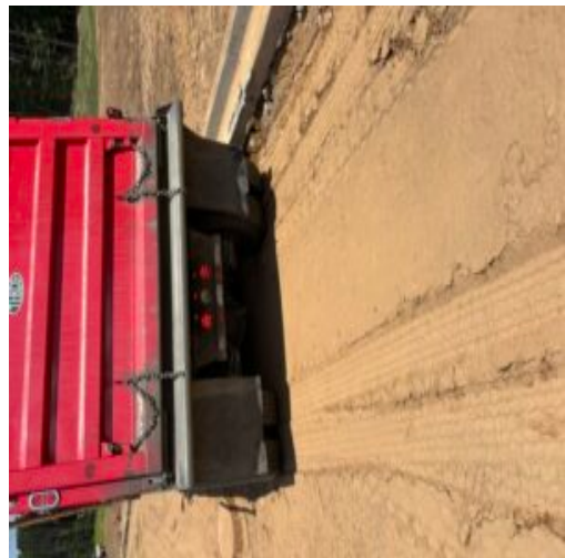
Proof rolling using tandem dump truck with 18.34 tons of base stone
