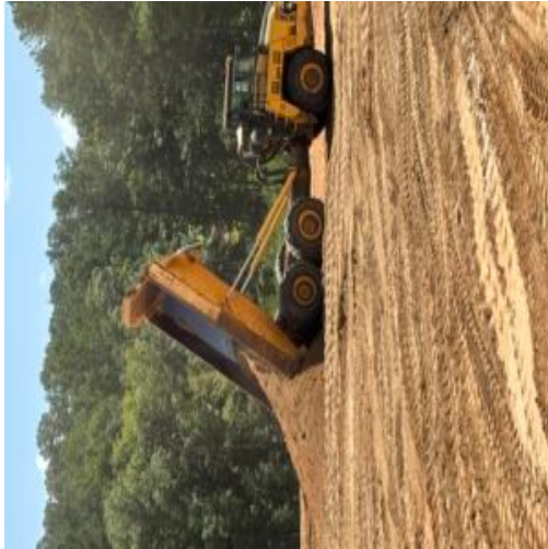
Fill placement at Shelly drive near detention pond
