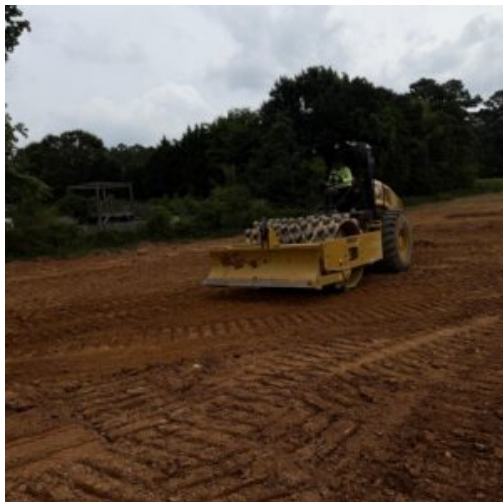
Compacting with sheep foot roller
