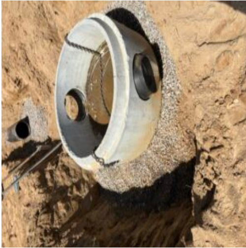
Installation of 12" sanitary sewer line between manhole #3 and 2
