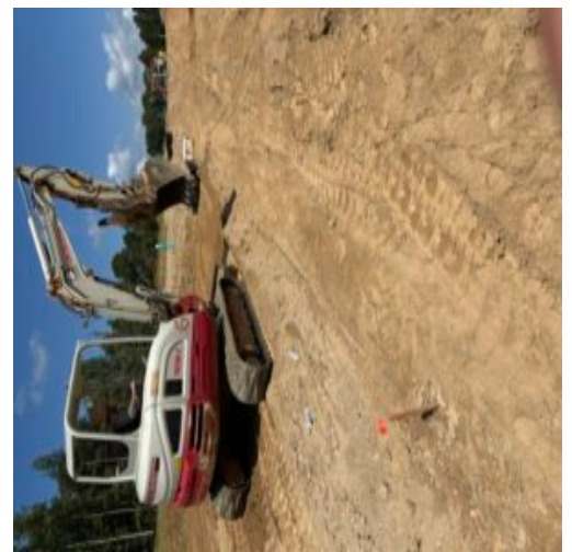
Installation of water lines and service meters without sufficient compacting efforts
