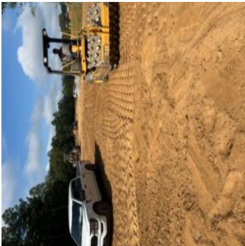
Installation of 12" sanitary sewer line between manhole #3 and 2
