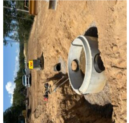
Installation of 12" sanitary sewer line between manhole #3 and 2
