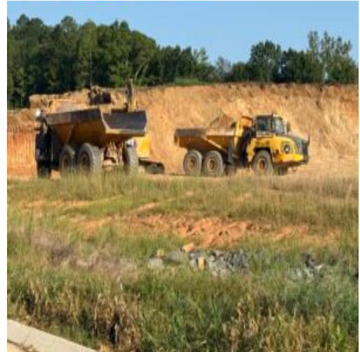
Cut area removing soil
