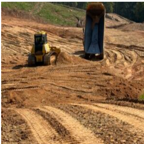
Backfill Road back of ammenities
