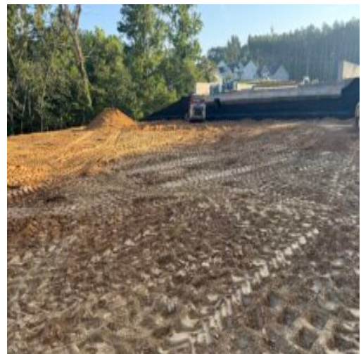
Backfill at bridge
