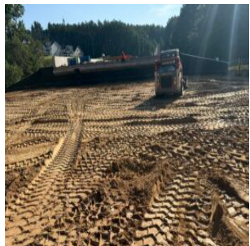
Backfill at bridge placement
