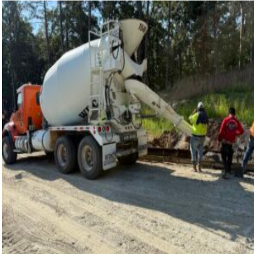
Wayne Davis Concrete used for Curbing
