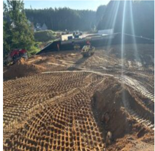
Backfill compaction at bridge
