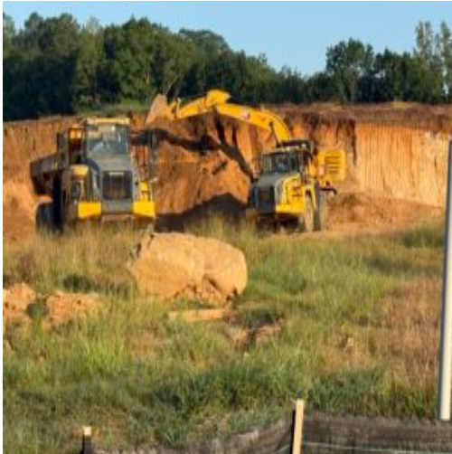
Cut area used for Backfill material of bridge
