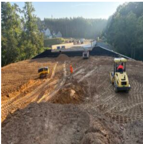
Placement of Backfill material at bridge
