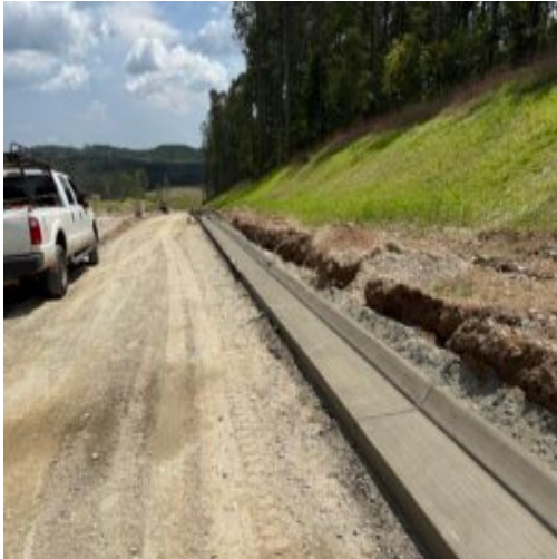
Daytime curbing placement
