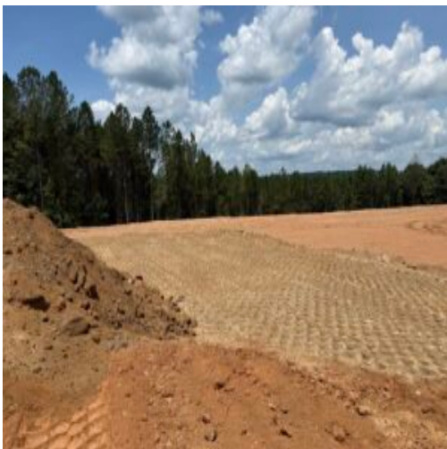
deep fill / backfill area for future development
