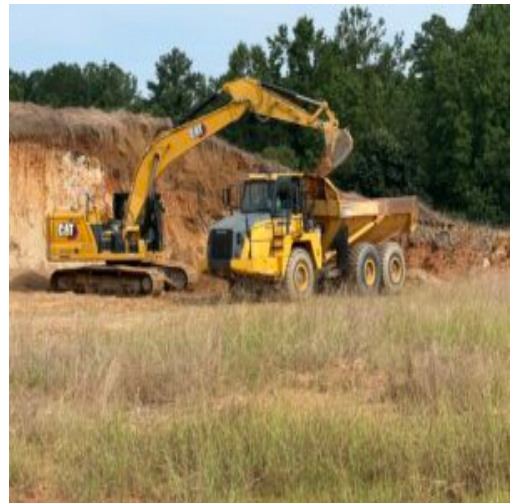
Material being loaded for bridge
