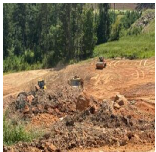
Working on slopes
