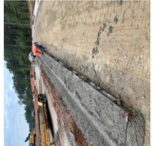
Observing pouring of 30"curbing at Nature Walk parkway
