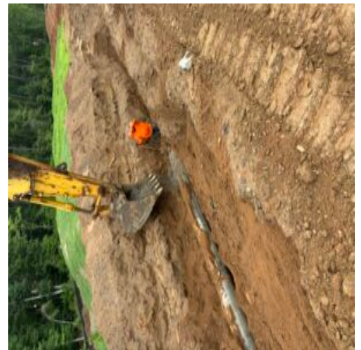
The contractor adding #57 stone under pipe after adjusting grade
