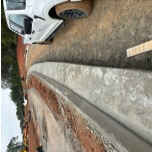
Observing pouring of 30"curbing at Nature Walk parkway
