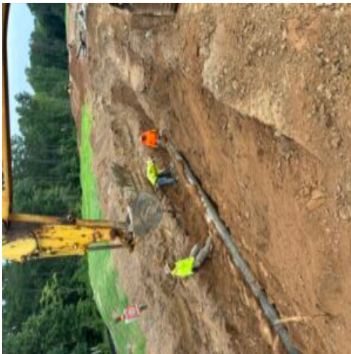
The contractor adding #57 stone under pipe after adjusting grade
