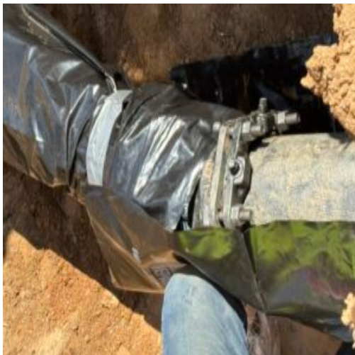
8" ductile water line double wrapped installed over gas lines.
