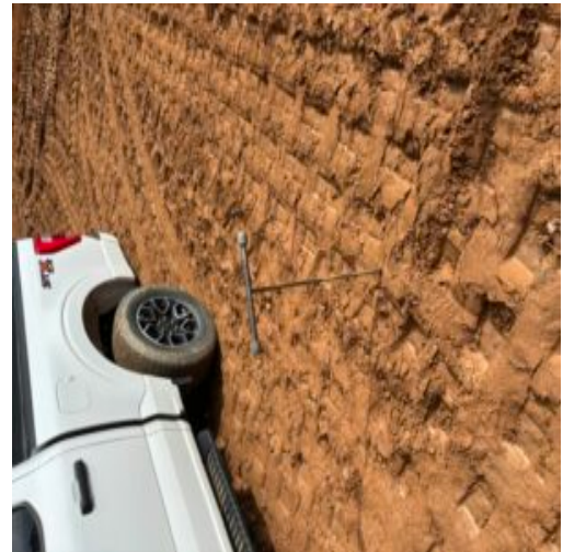
Probing in place fill at lots 33 and 34
