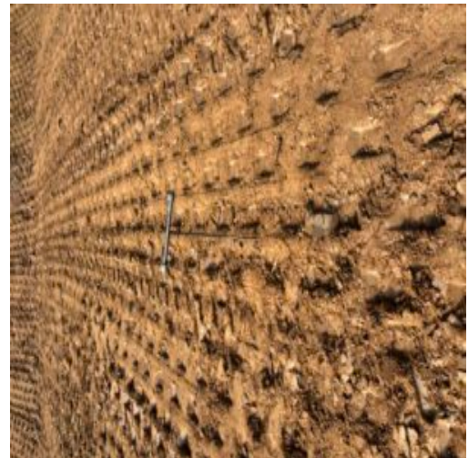
Observation of existing sub grade at lots 33 and 34.
