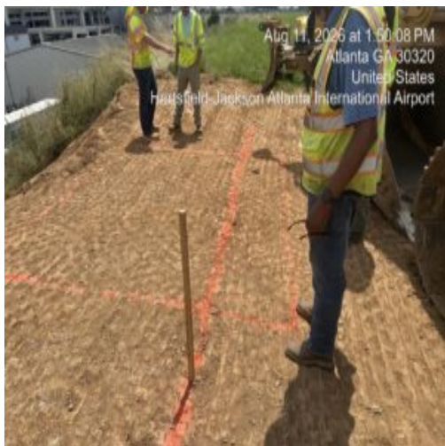
Marked area to excavate
