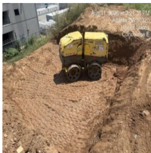
compacting excavated area using trench packer.
