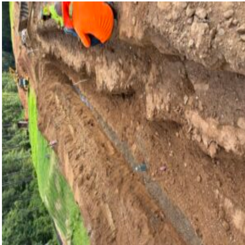
Excavated trench for 16" casing for sanitary sewer line placed on # 57 stone.
