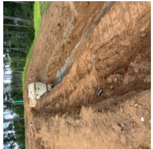
Excavated trench for 16" casing for sanitary sewer line placed on # 57 stone.
