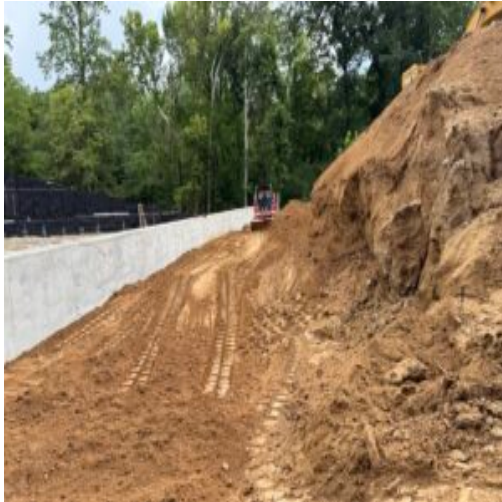
support retaining wall
