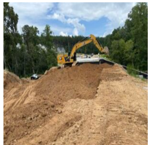
Excavator moving soil
