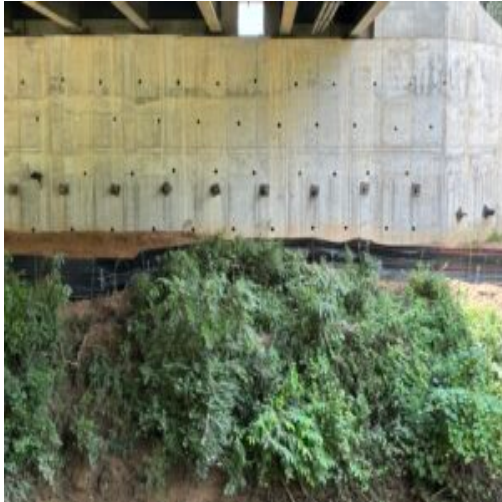
Tension rods observed at abutment wall
