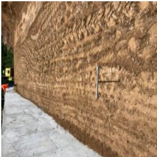
Recommending additional compacting efforts at wall backfill
