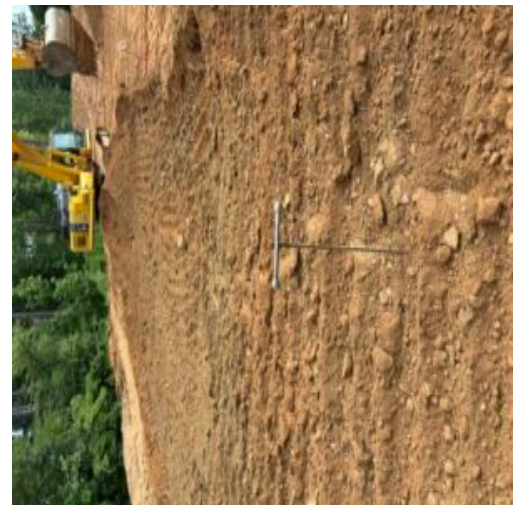
Observation of subgrade after removal of in place saturated fill soils, approved for additional fill placement
