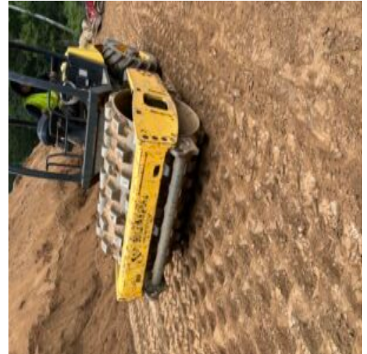
Compacting fill at dead man footing wall
