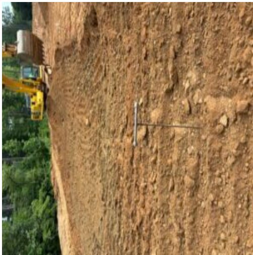
Observation of subgrade after removal of in place saturated fill soils, approved for additional fill placement
