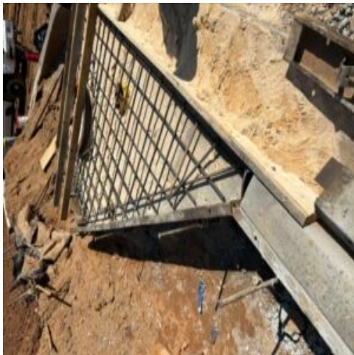
Observation of reinforcing steel at curb inlet throats
