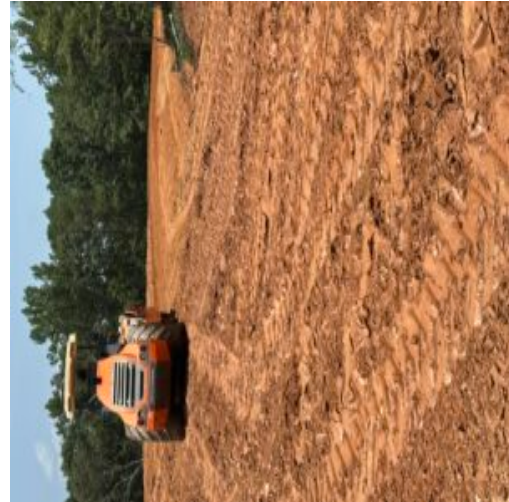
Fill placement at Unit 4 phase 3 to re compact and test at later date.
