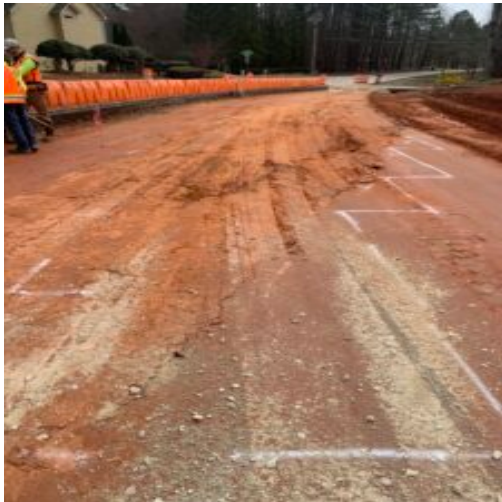
Subgrade proof-roll between Sta 0+00 and 5+00
