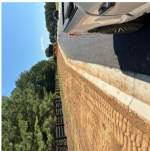
Sub grade prep. at deceleration lane on Seven Hills side walk
