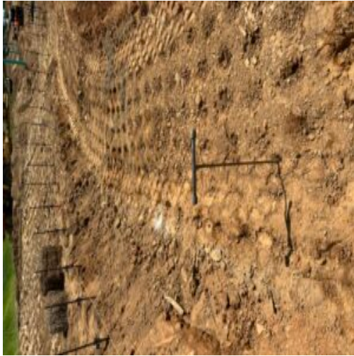
Probing sub grades at roadway curbing with estimated compaction efforts of 90% to 92%.
