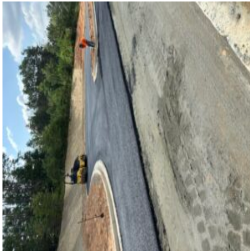
Placing 19mm asphalt binder mix
