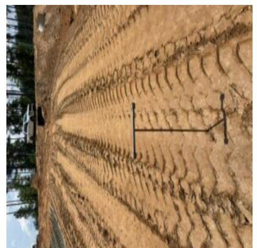
Probing in place compacted fill after mixing and compacting in the static mode
