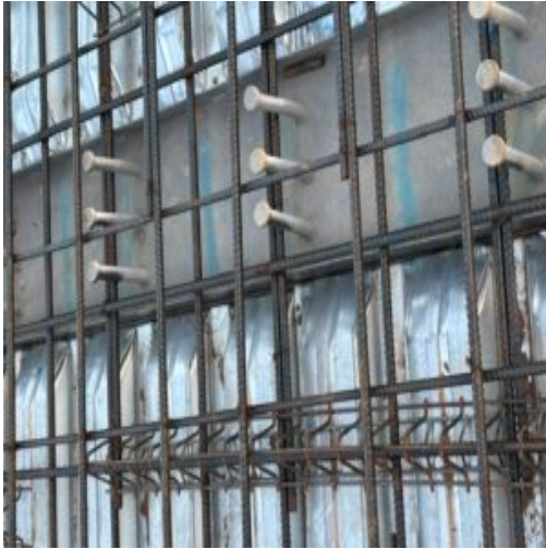
Resteel observations panel decks were cleaned
