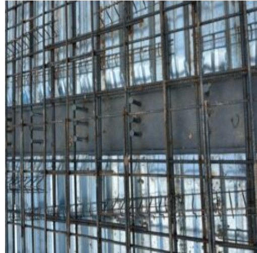
Observation of reinforcing steel in place at bridge slab panels according to site document in title Bridge Deck,dated 2/20/26.Drawing No. R3.0
