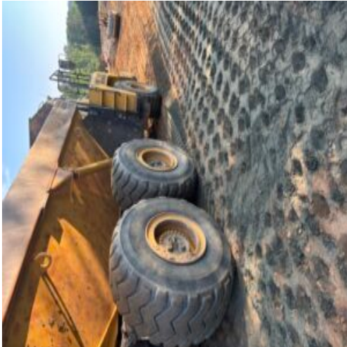
Fill placement and compacting efforts at roadway over gas line.
