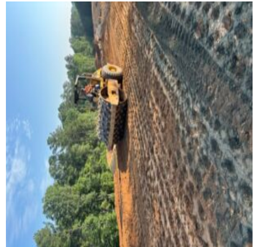
Fill placement and compacting efforts at roadway over gas line.
