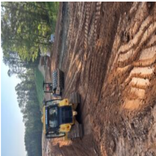
Fill placement and compacting efforts at roadway over gas line.
