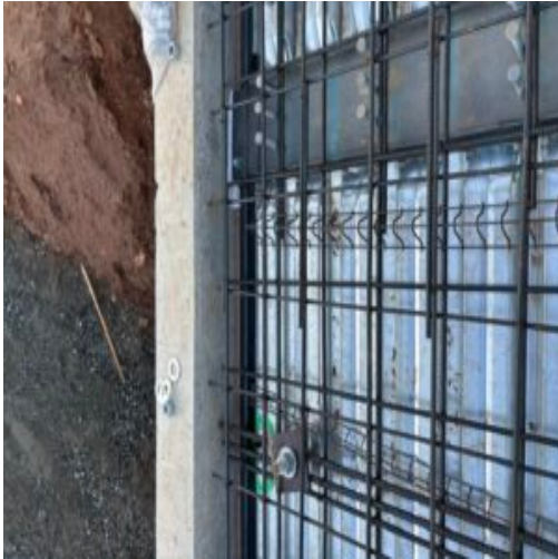
#6 vertical bars in place at support dowel rods manhole # 12 which clipping was recommended to repair from rain events and construction traffic
