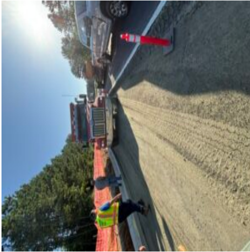
Sub base proof roll at decel. lane and roadway being observed by Paulding County, J&W Paving and Thompson Grading
