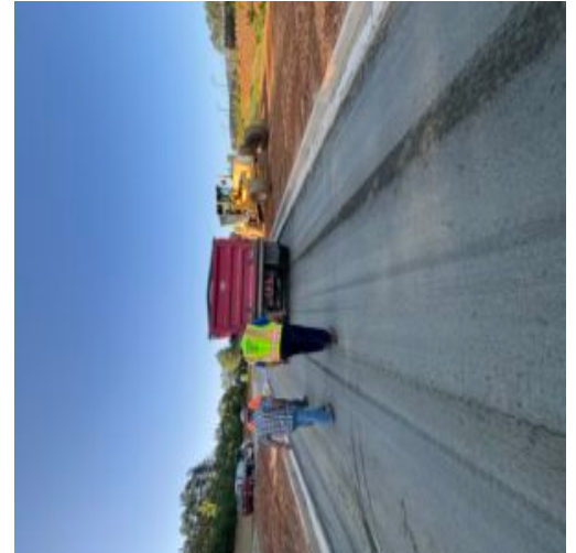
Sub base proof roll at decel. lane and roadway being observed by Paulding County, J&W Paving and Thompson Grading
